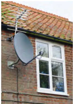
Satellite dish, aerial and uPVC window
