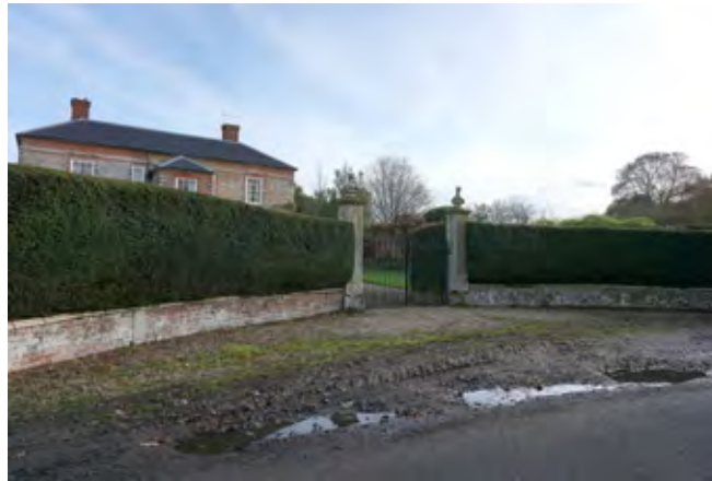
Grade II listed gates to the Manor House
