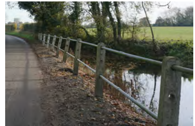
Concrete post and steel pole fence, which is not in keeping with the character of the village
