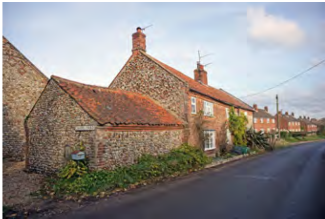
Cottages on The Street
