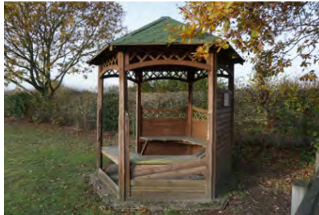
Damaged shelter at the playground
