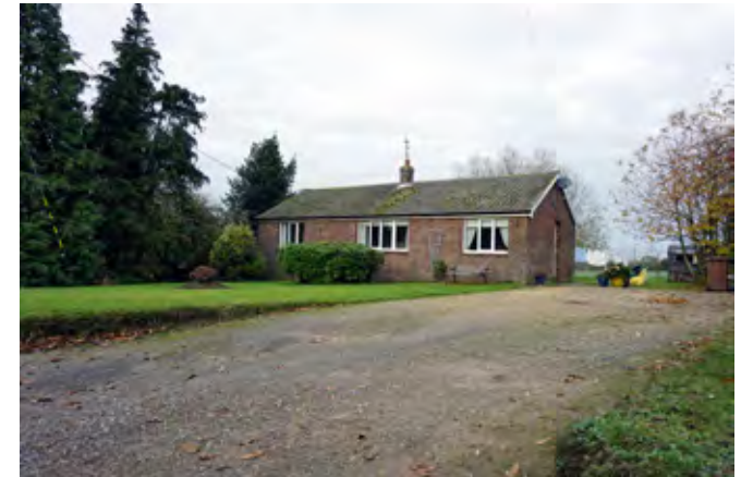
Mid-late-twentieth century bungalow on The Street
