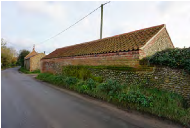
Farm buildings on The Street
