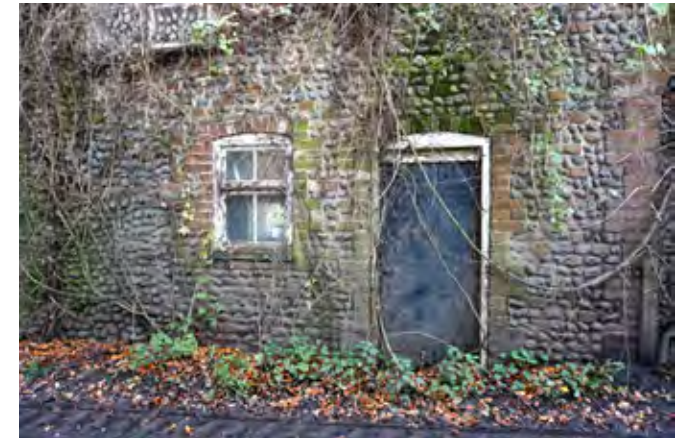
Timber work in poor condition
