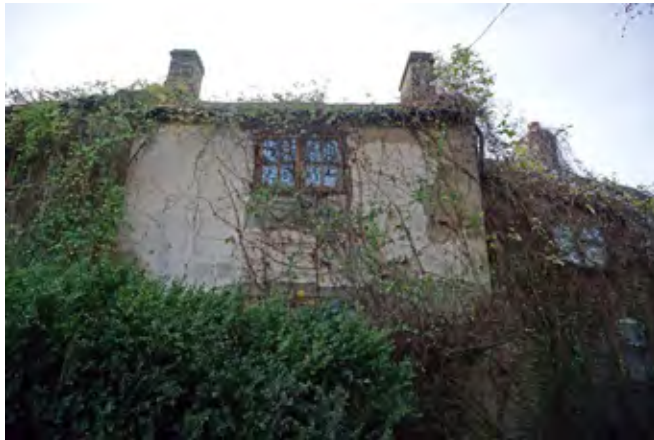
Cementitious render repairs
