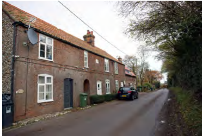
Terrace of cottages on The Street dating from 1890
