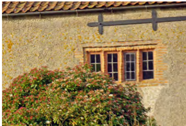
Brick mullioned window on the farmhouse at Pitt Farm which stylistically dates to the 16th or 17th century
