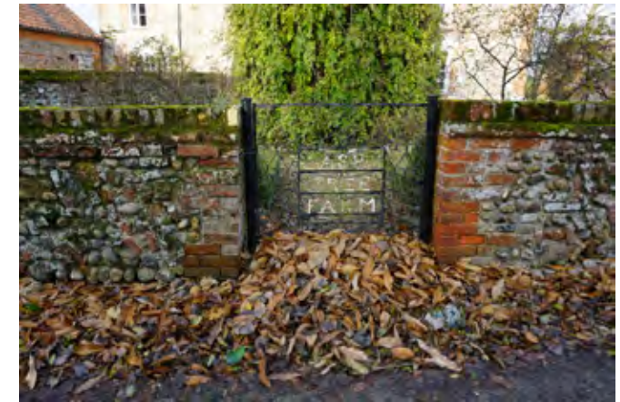
Brick and Flint wall with decorative metal gate to Ash Tree Farm
